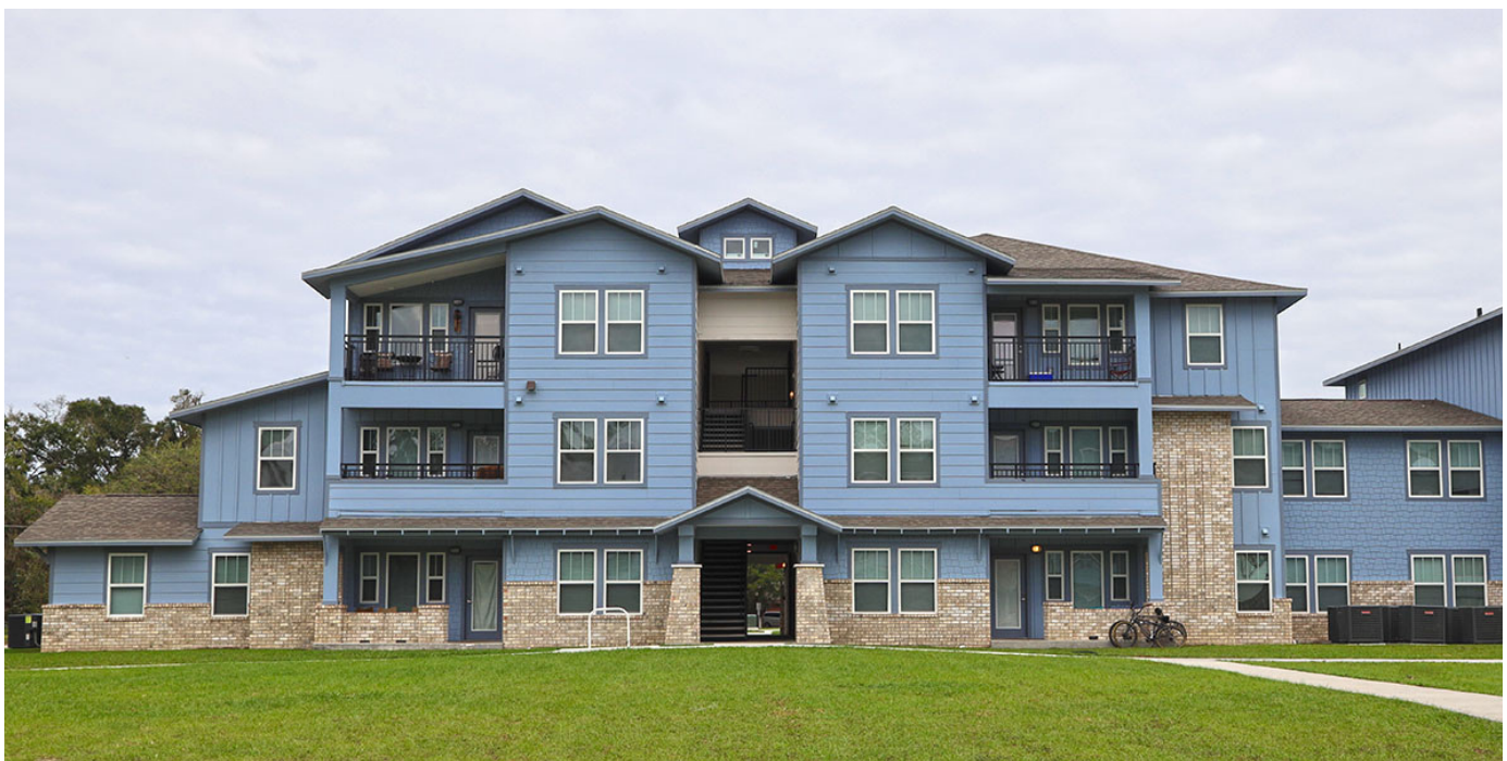
Gainesville Housing Authority: Woodland Park Phase I
