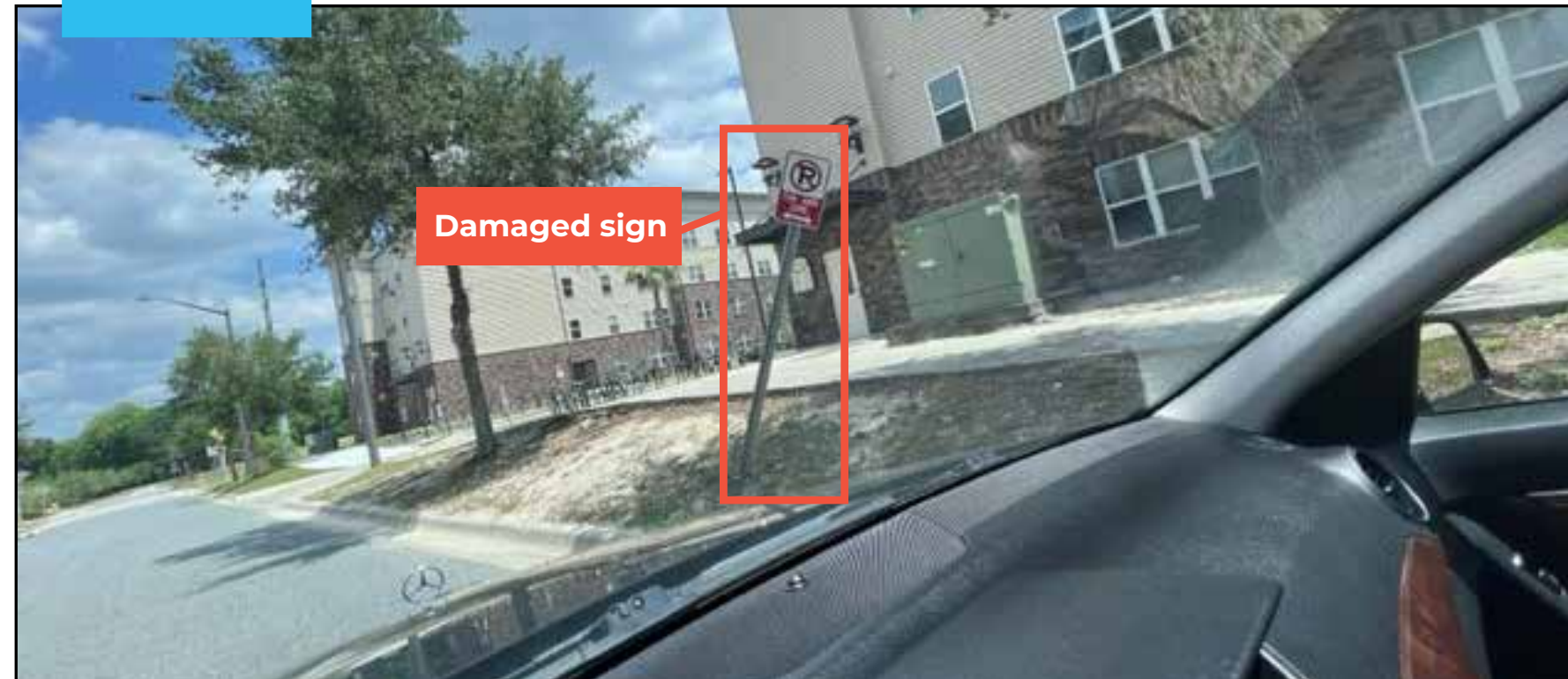
Damaged sign at SW 37th Street.
